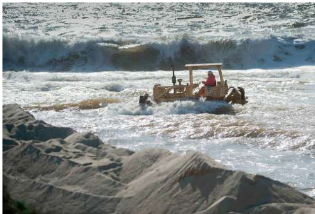
Second Place - Diverting Carmel River at Flood Stage (2) Jeff Hobbs
